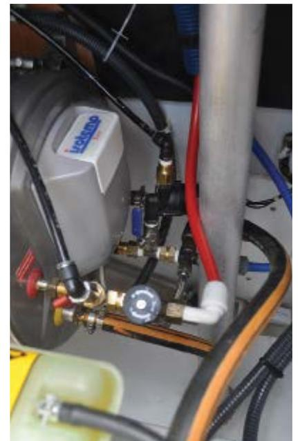
Stop the cold supply and connect the return line to the hot side: turn on the cold supply and bleed the system of air, usually at the highest point at the panels. Turn on a hot tap to bleed the hot circuit of any air and to ensure the reservoir is full.
